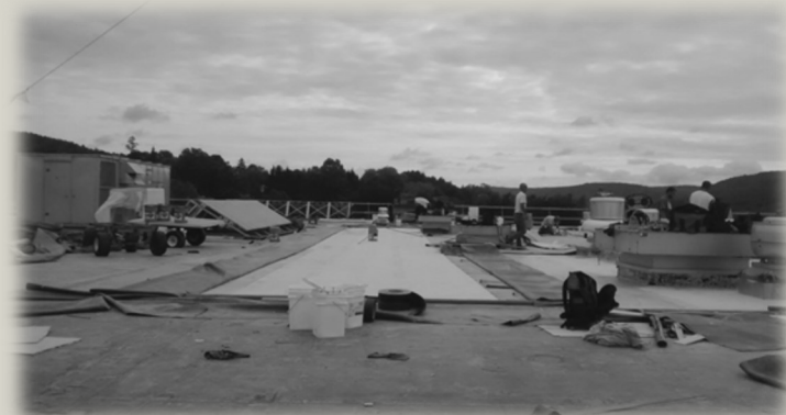
High School Roof Project
